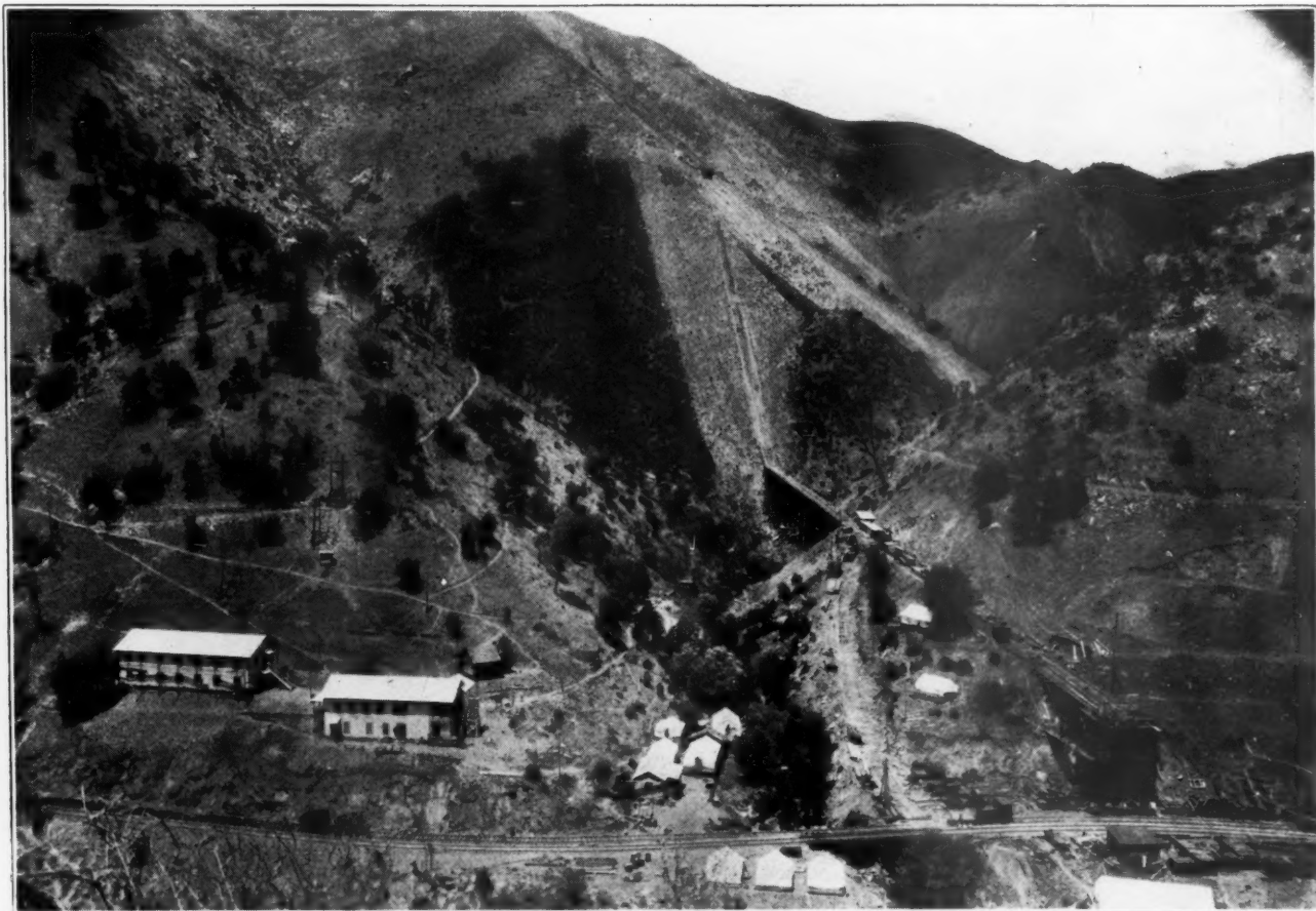
Unusual Deposit. Quarry incline, railroad, storage bins and quarry in upper center
